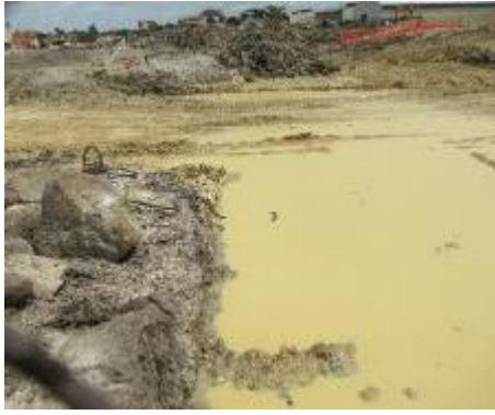
Image: Poor site management results in sediment laden stormwater making its way into creeks.
